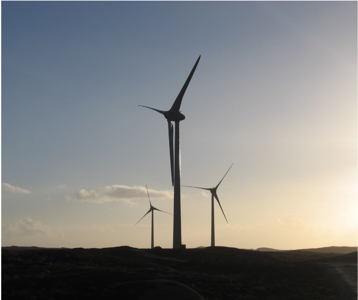
Photo - Lochcarnan Community Windfarm, part of the 93,000acre community owned Stòras Uibhist estate, South Uist.
